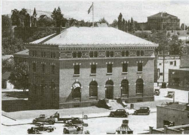
Old Federal Building - Corner of 2nd & Washington Sts., looking Southeast.
