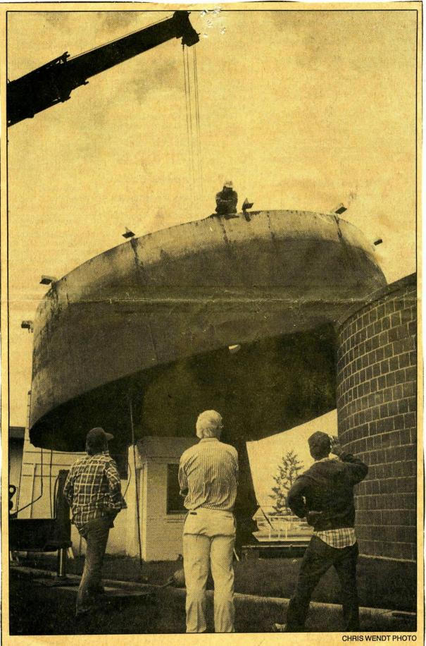
OOPS: Plant workers at the Moscow wastewater treatment plant had a busy Monday, when a crane tipped over trying to lift a 10-ton dome lid from the plant's secondary digester tank. The lid landed on top of the tank, and on a nearby storage building. Assistant city engineer Dean Weyer (center) is shown here helping employees of Wilbur/Fletcher Inc. of Dayton, Wash. — the crane operators — lift the tank top, which was eventually put on the ground for repairs. No damage estimates are available.
