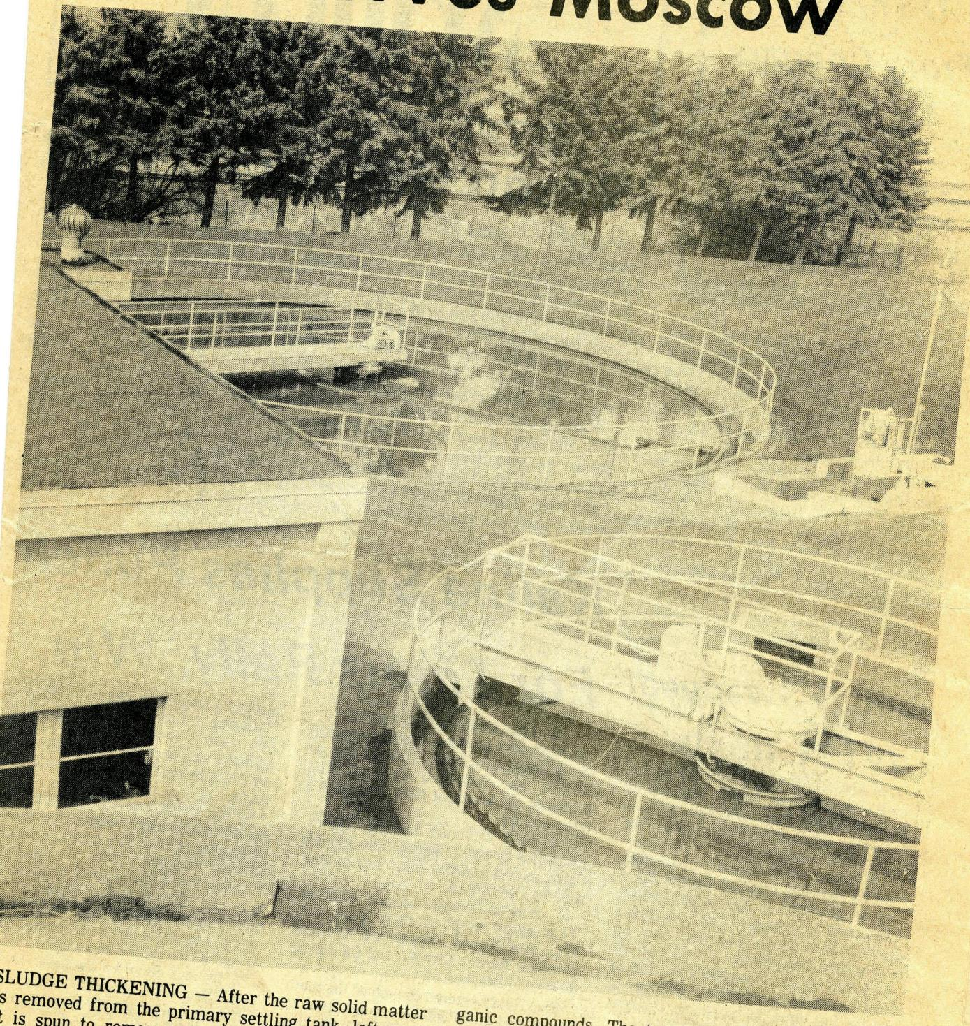
SLUDGE THICKENING — After the raw solid matter is removed from the primary settling tank, left rear, is spun to remove grit and pumped into a sludge nickening tank, foreground right, where solids settle the bottom and water flows through seine teeth over it is pumped to a large digester. In the digester anerobic bacteria to on the organic matter, and reduce it to stable or-
