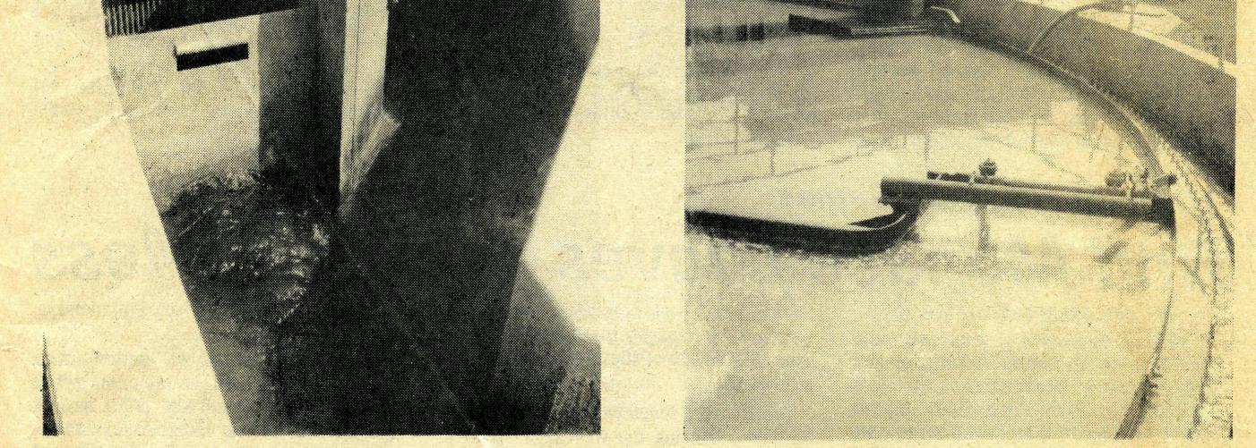
SEWAGE CHOPPED, SETTLED, AND SKIMMED – Raw sewage entering the plant is chopped, and all rags, golf balls, wood, paper, and other items reduced to small particles that will not clog the system. Shown left is the chopping operation with raw sewage entering the plant. After chopping the sewage is pumped
