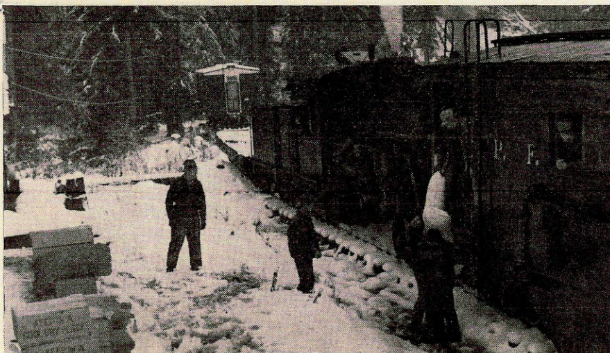
Unloading supplies at Camp 14 when the PFI train made its last trip in for the winter.
