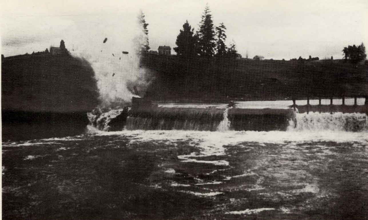
After the jam formed, it had to be broken up by blasting.
