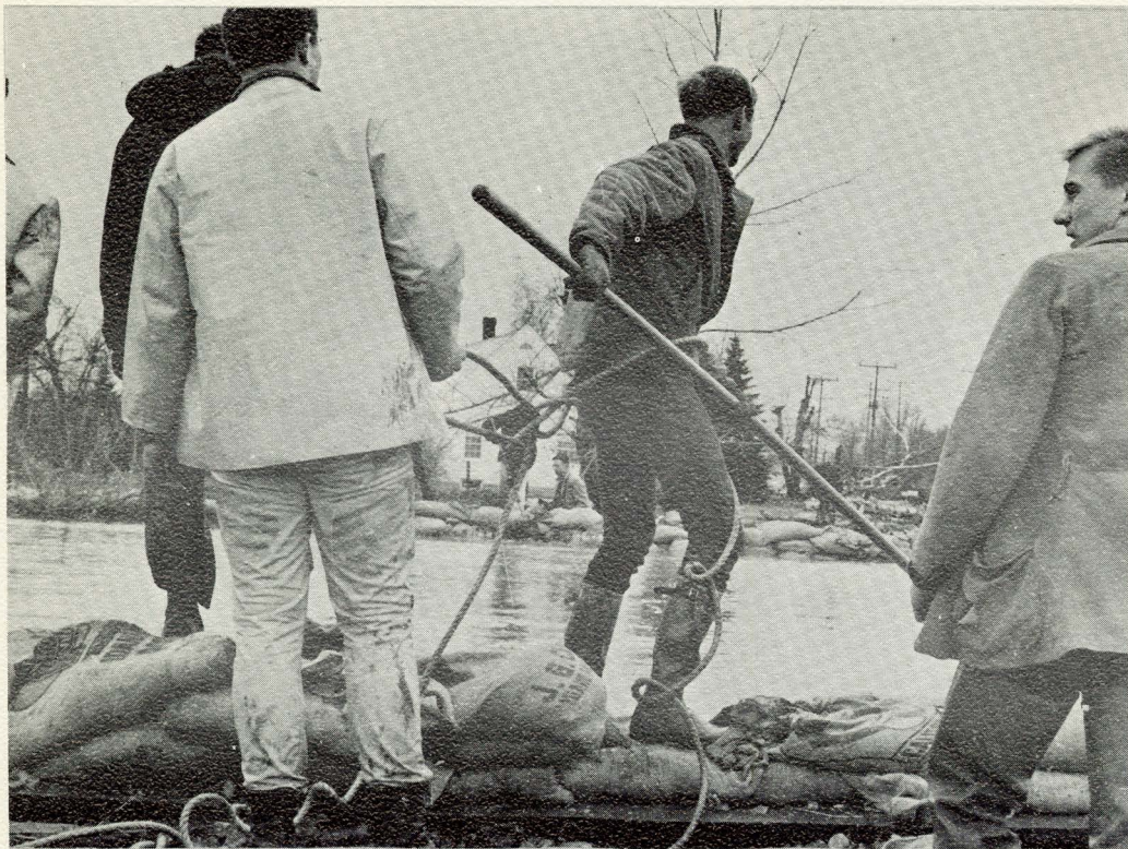
Long poles were used to snag pieces of ice before they got hung up on a bridge. And just in case a piece of ice in return didn't snag a man attempting to snag it, a rope around the waist was used. At 15th and Emerson the water started running over the bridge so men quickly built a sand bag dike.
