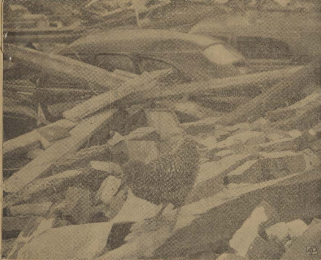
This lonely chicken, who came through the death-dealing tornado unscathed at Albany, Ga., surveys the wreckage left by the blow. The twister clipped trees and shattered buildings, causing such shambles as are shown here. Early reports listed 23 dead, about 500 injured and property damage at between 5,000,000 and $9,000,000.
