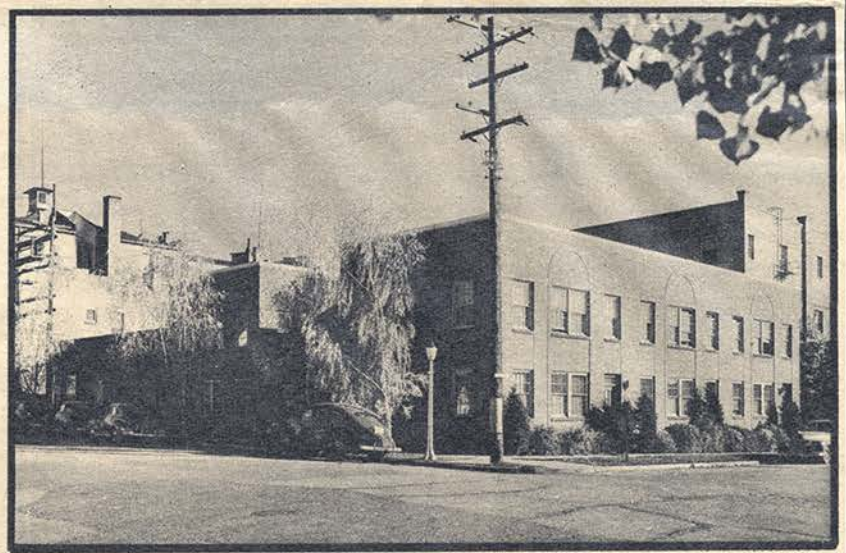
THE PROFESSIONAL BUILDING , Moscow's largest and most modern office building, is owned by Dr. Robinson and is tenanted by doctors and lawyers. The Psychiana Building, also owned by the Doctor, is right next door.
