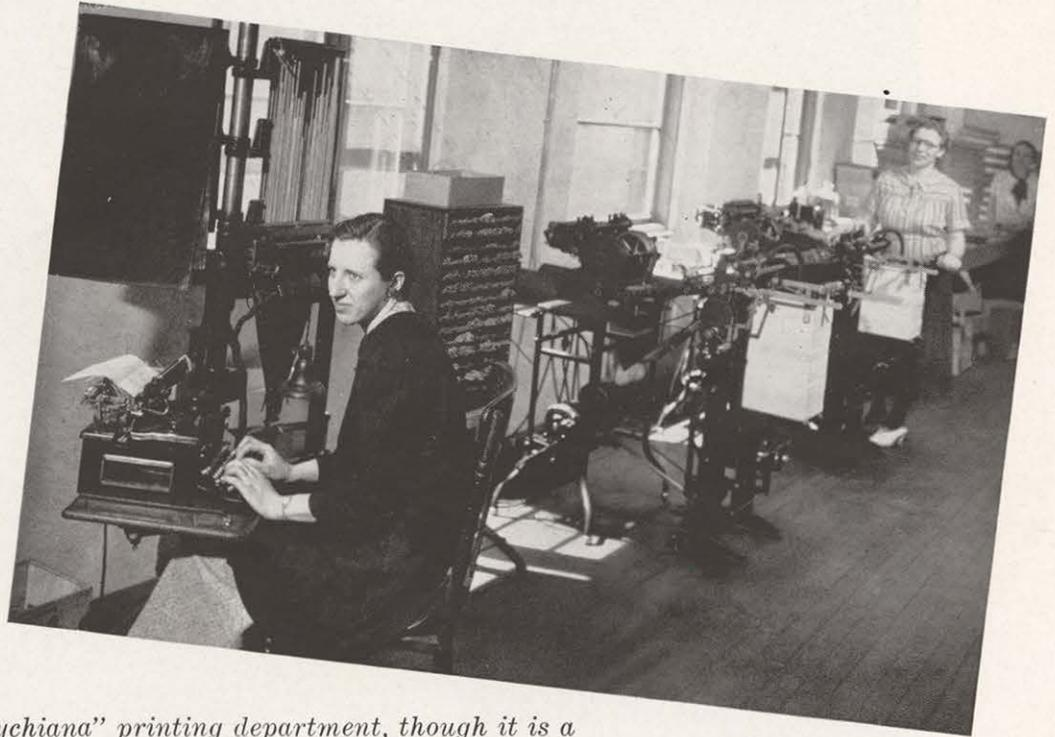
*This is a picture of the "Psychiana" printing department, though it is a small part. Two fast multigraph machines and a double size multilith are employed, and these three machines, working 24 hours a day, can produce half a million printed sheets, 8½ by 11. The "Psychiana" plant is equipped to receive as high as 500,000 replies daily, mailing all mail to those replies inside of 24 hours. The whole plant runs like clock-work. It is one of the most highly efficient plants in America.*
