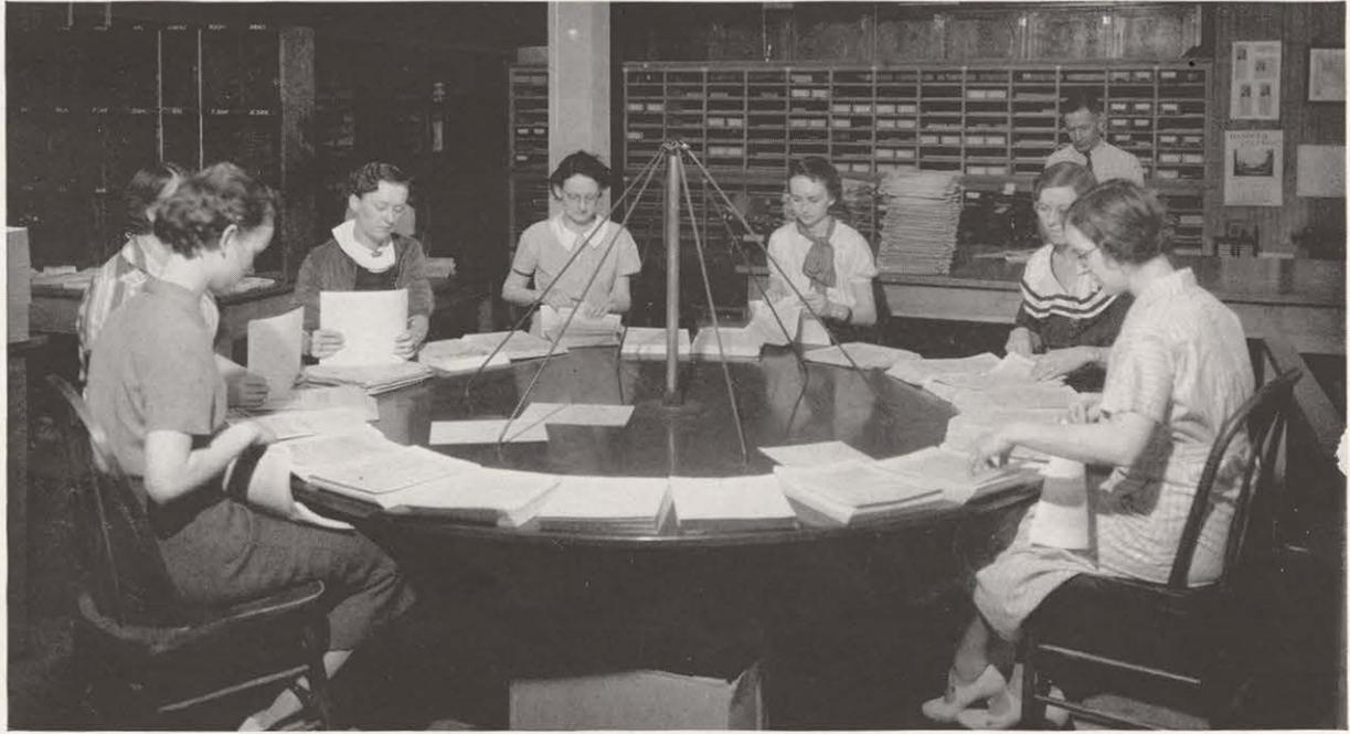
*This is a revolving table used in the assembling of the literature. Eight girls can sit at this table, and in one hour, enough of each Lesson or follow-up can be assembled to suffice for that day. The table revolves by underneath motor.*
