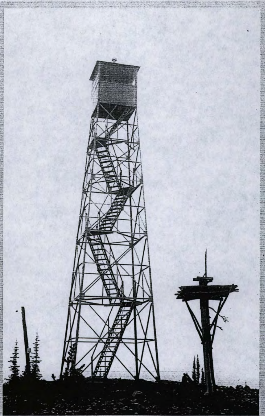
Pl. 4-c The 60 foot-high tower was sited a short distance west of the cabin. The 9x9 foot room at the top of the tower was accessed through a trapdoor in the floor.
