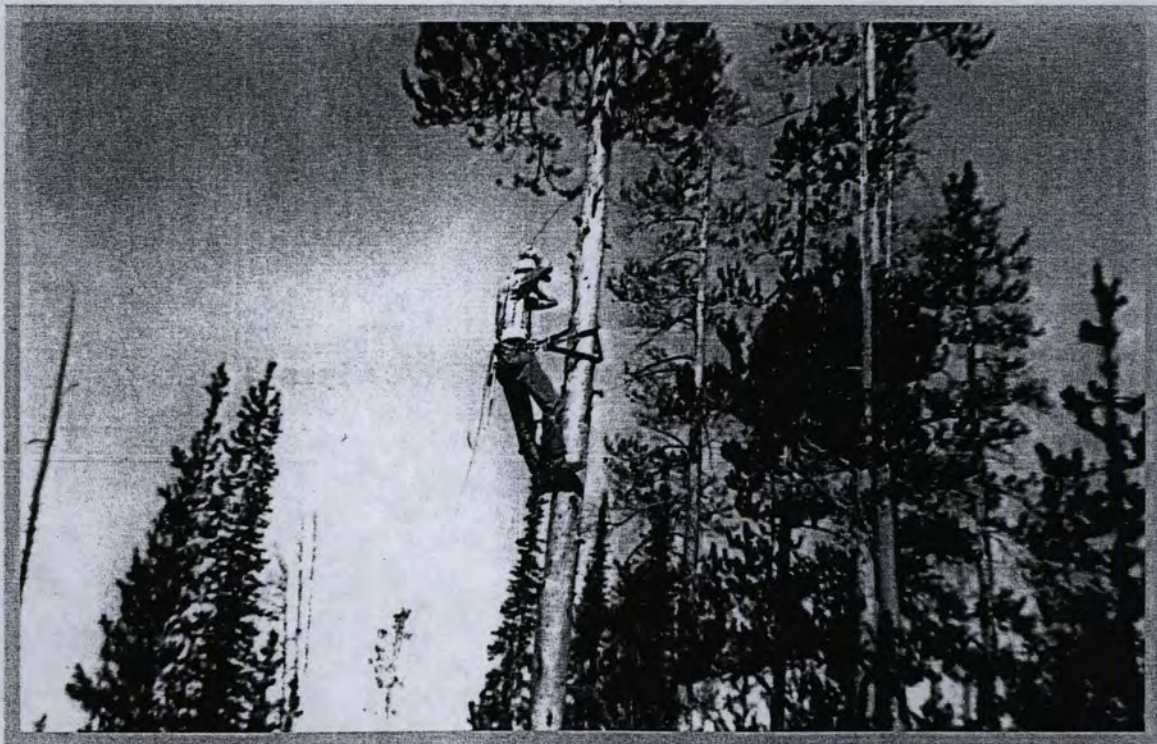
Pl. 5-b Bob Dustman repairing a telephone line.
