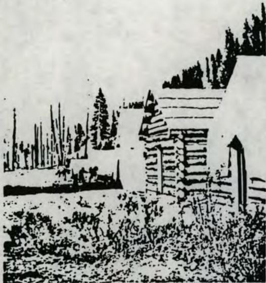
Roosevelt under construction, 1902. Note the Mining Recorders office in the right foreground.
