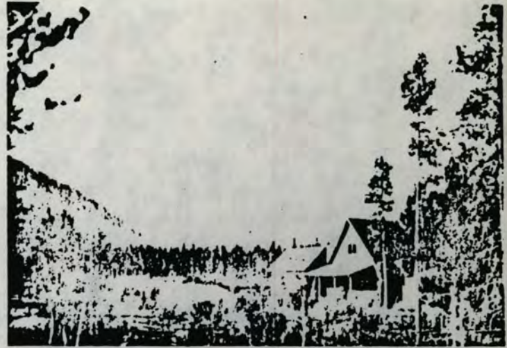
Edwardsburg as it looked in the early 1900's. Looking up Big Creek in the direction of the Belvedere area and Profile District. These historical structures are still standing.
