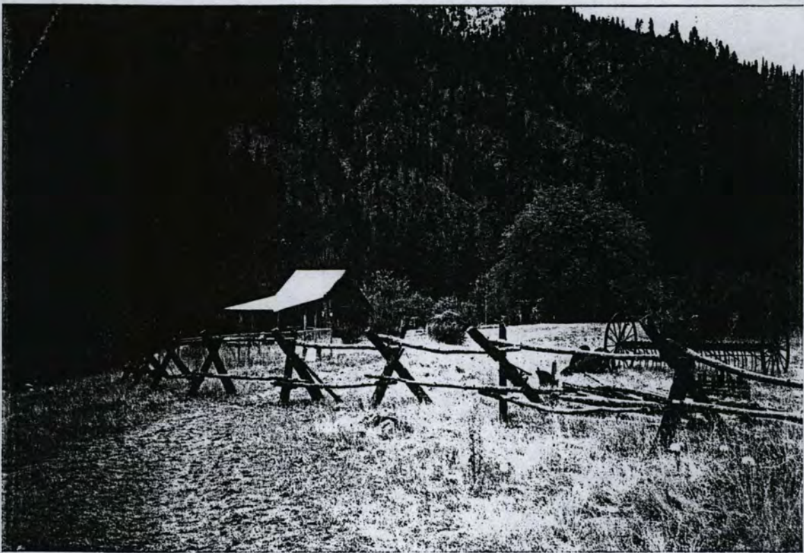
STABLE, WEST OF DWELLING WHICH IS HIDDEN BY LARGE TREE (PRESTON PHOTO, 2000)
