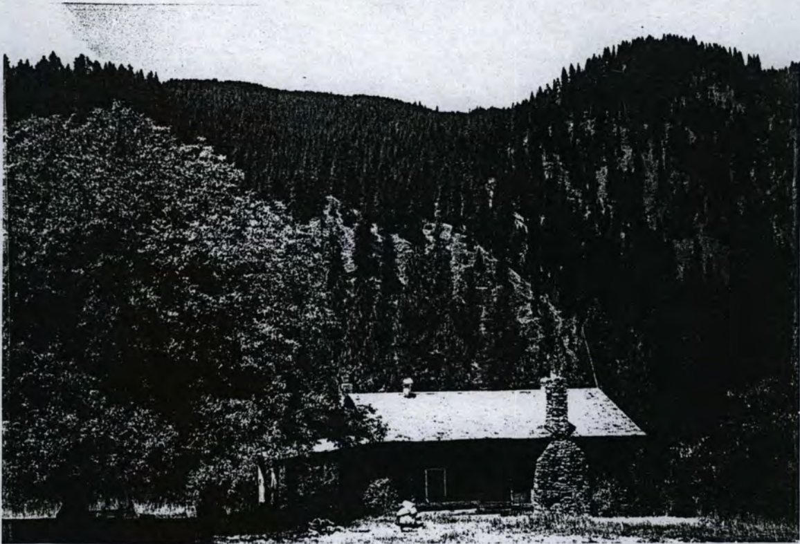
CAMPBELL'S FERRY DWELLING, LOOKING WEST TOWARD SALMON RIVER (PRESTON PHOTO, 2000)
