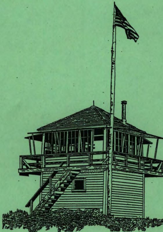
INDIAN MOUNTAIN FIRE LOOKOUT BUILT BY THE CCC'S IN 1933
