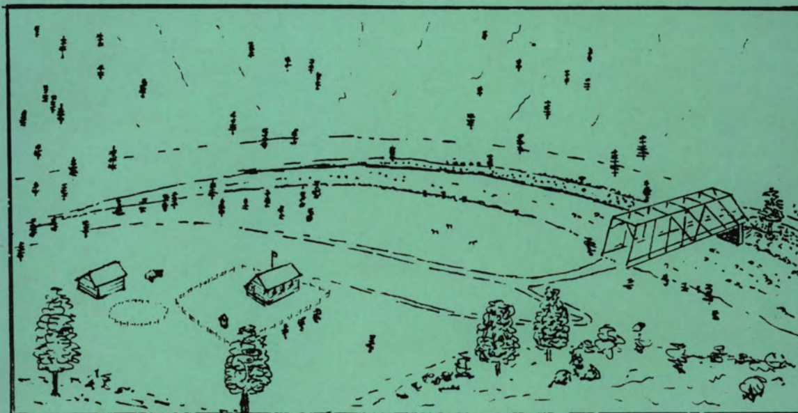
SOUTH FORK GUARD STATION AND DUSTIN BRIDGE, C.1929
