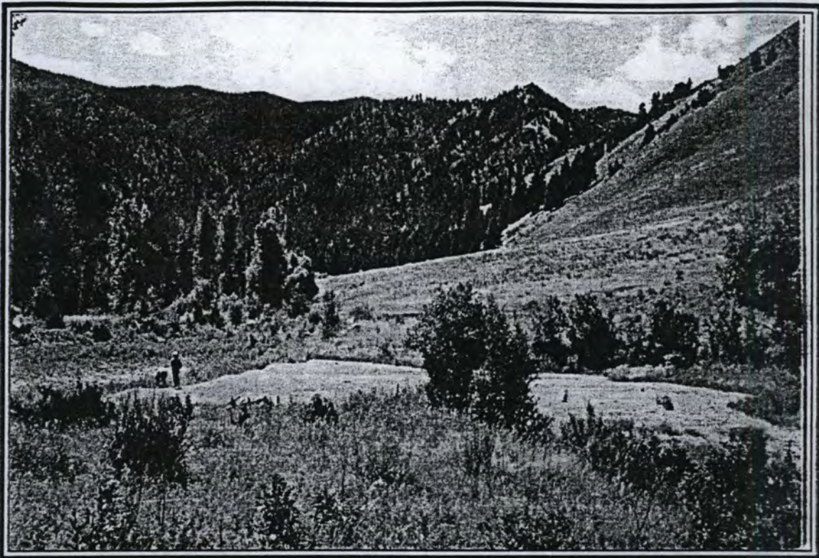
Figure 7. Deposition of sediment in abandoned reservoir as a result of the overland flow of Cow Creek.
