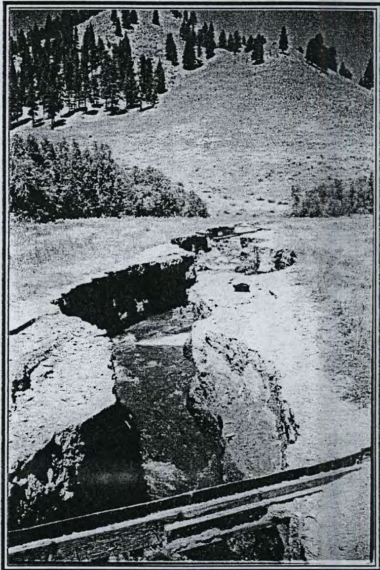
Figure 1 Gullied Cabin Creek airstrip.
