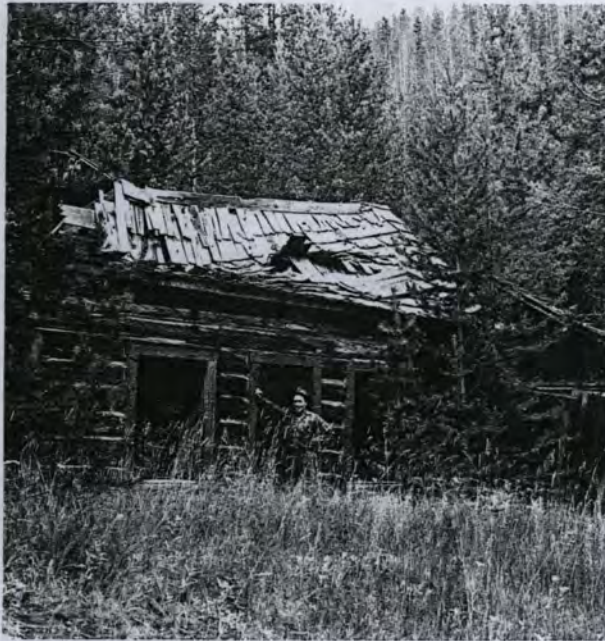
The substantial cabin of a miner survived many winters near Cobalt
