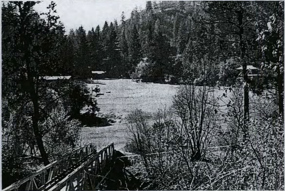
BRIDGE OVER BIG CREEK
