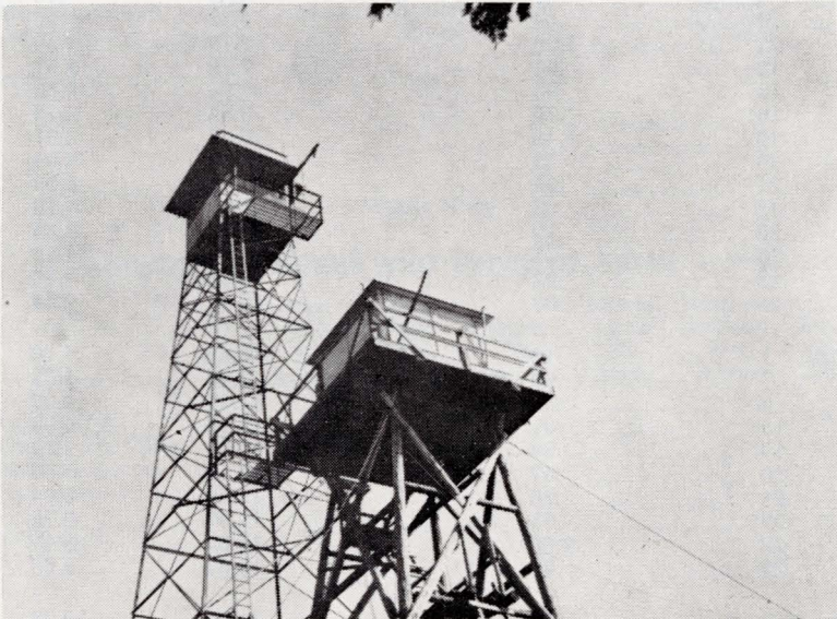
New steel tower on Elk Butte with old wooden tower in foreground.
