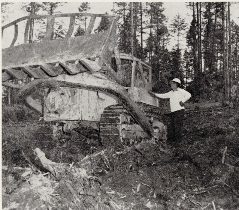
Emil Keck, chief slash disposal supervisor and assistant fire warden, instructs operator on use of new 1950 model D6 tractor equipped with specially built and improved brush piling blade.
