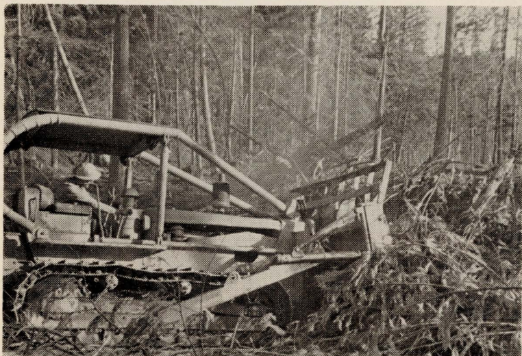
DOZER PILING BRUSH
