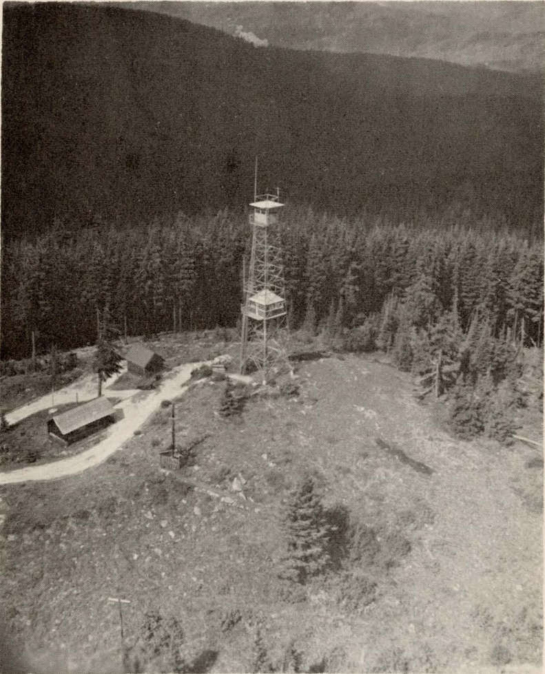
This modern new steel tower at Elk Butte lookout is the key to our detection and communications facilities. A power line is built to the location to provide the modern conveniences necessary. If the five mile power line fails emergency power plant takes over.
