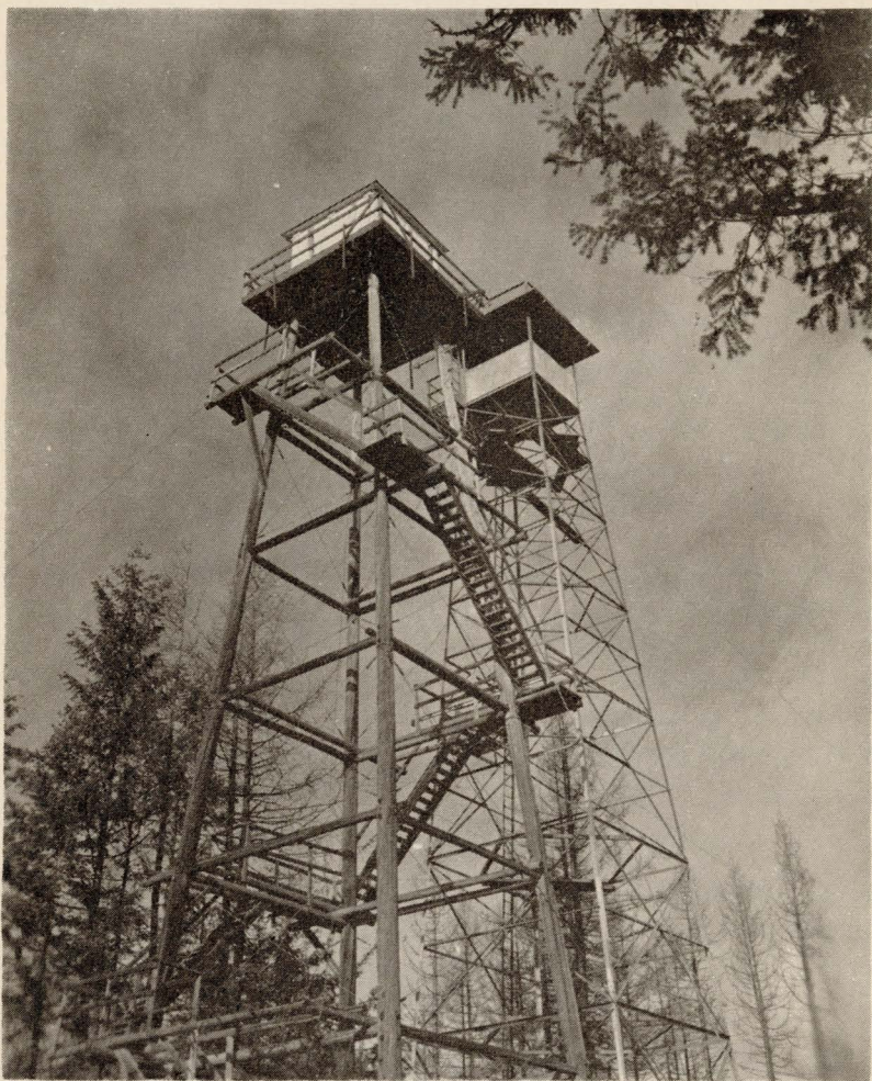
Mason Butte lookout built in 1934 with CCC help was replaced in 1962. The new steel tower (right) was purchased from war surplus stocks. While its design was made for aircraft spotting work in the South Pacific, bullet proof and all, it will serve for many years to protect the forest from fire.
