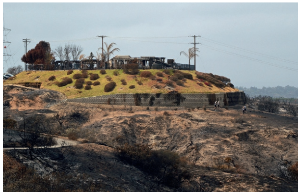
FIGURE 13.2 Homes burn because they are flammable. Many homes with adequate defensible space still burn in wildland fires because embers land on flammable materials around the home or enter through openings such as attic vents. These two homes burned during the 2014 Poinsettia Fire in Carlsbad, California, despite fire-safe landscaping, a firewall, and thinned wildland vegetation. Focusing exclusively on wildland vegetation clearing ignores the main reasons homes burn: they are flammable. (Photo credit: Richard W. Halsey.)
