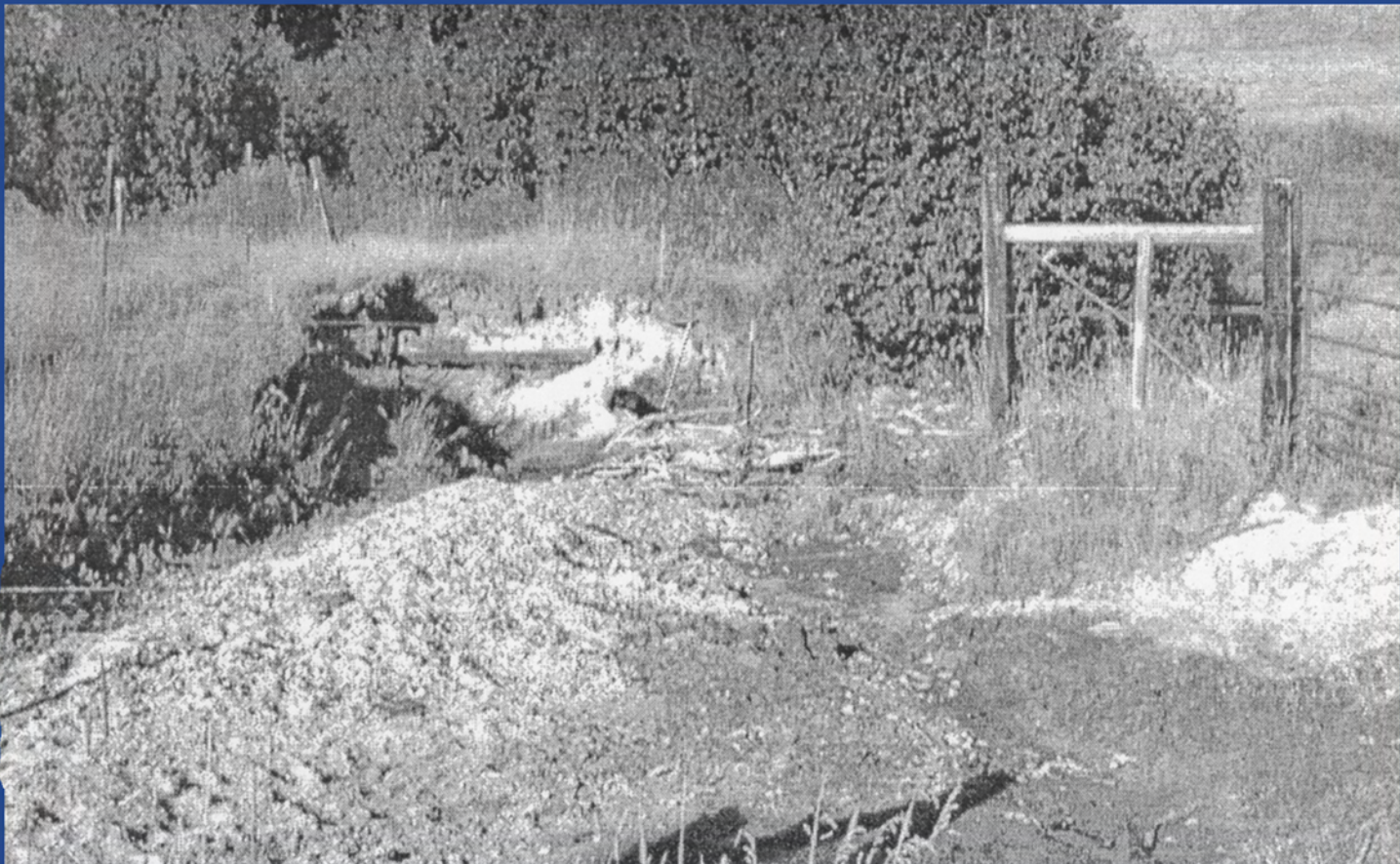
Figure 5: East Hatter Creek stream crossing showing sediment accumulation
