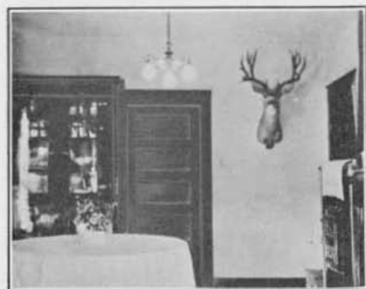
The residence lighting is provided by centrally located cluster fixtures
