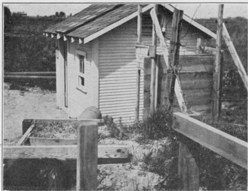
The Franklin Road drainage plant showing discharge pipe
