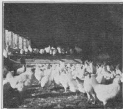
View of poultry water heater installation
