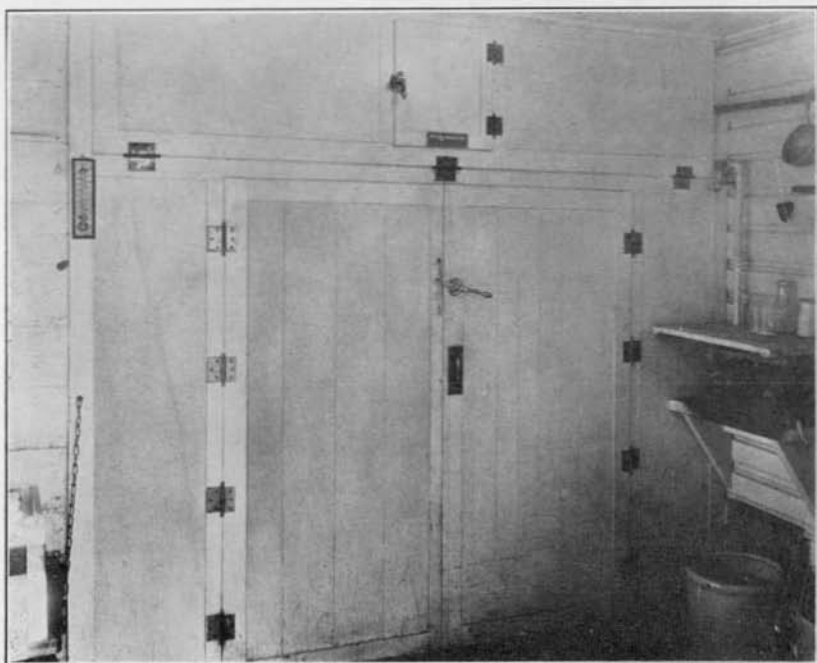
Cold storage box for commercial dairy installation located near Moscow
