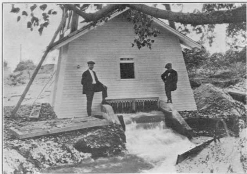
Orchard Avenue Pumping Plant—No. 1 of the Pioneer Irrigation District
