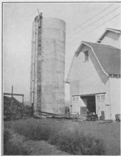
Silo filling with electric motor power
