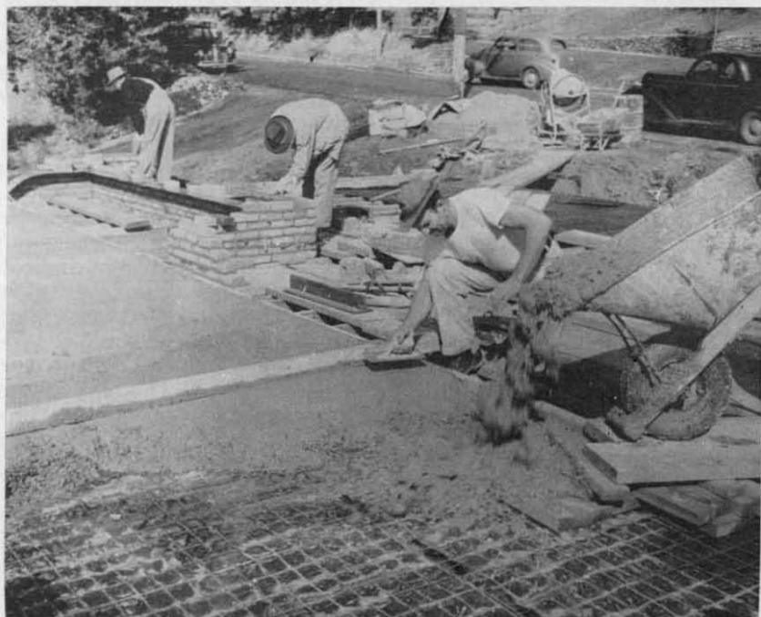
Figure 5.—Pouring wood-waste concrete floor in a Moscow residence.
