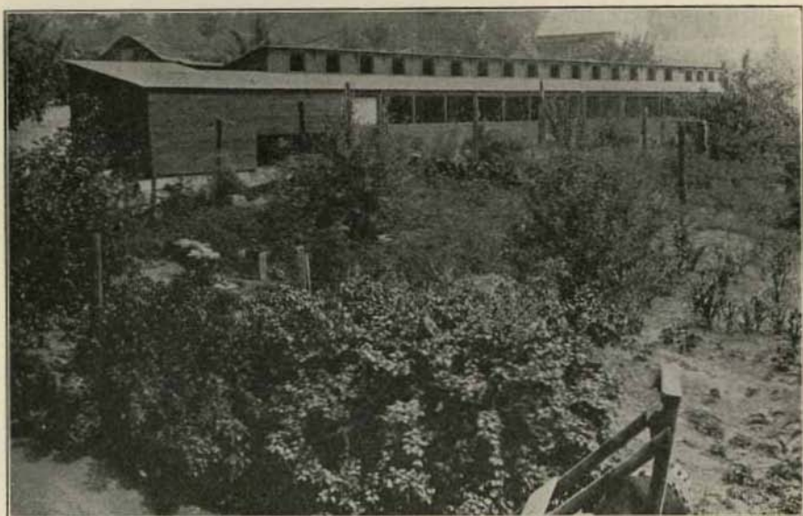
Fig. 3. A Shed-type Remodeled to Conform to the "Idaho Model Half-Monitor" Poultry House.
