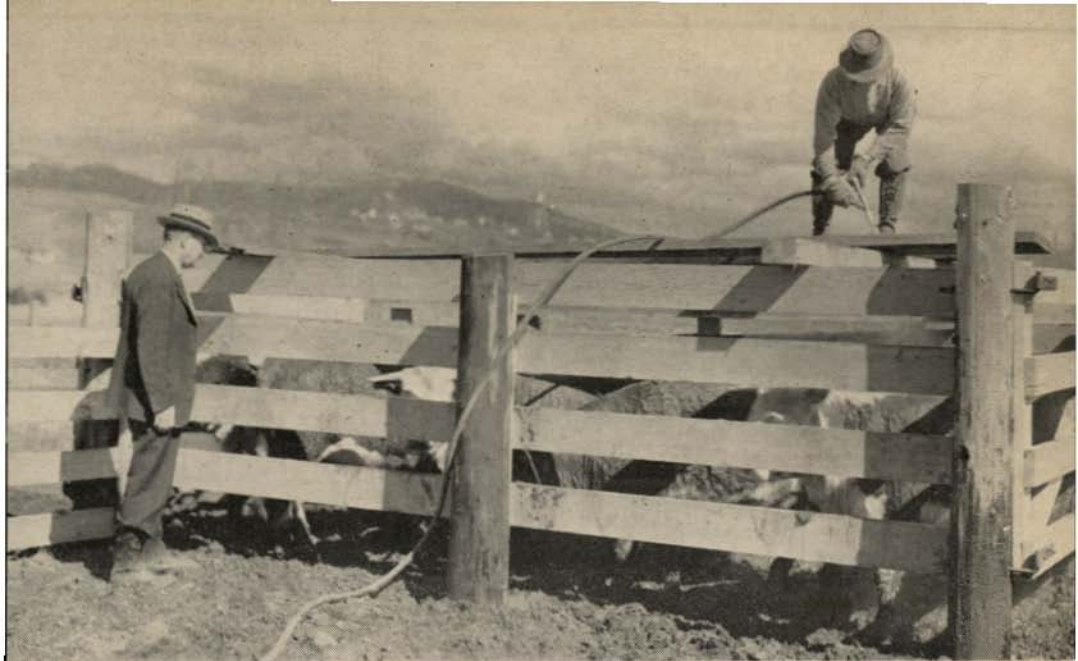
Figure 7.—A small spray corral made of planks and posts. Note the operator is too high above the animals.
