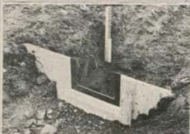
Looking upstream on installed weir. Note the gravel and rock protecting apron and the staff gauge location
