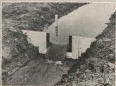
Looking upstream on installed weir. Note the gravel and rock protecting apron and the staff gauge location
