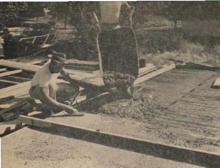
Pouring a floor slab of light weight concrete. The steel-text on which the concrete is poured serves as a form and for reinforcement.
