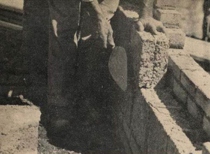
Laying precast blocks of S D concrete. Blocks were laid as back-up for the brick veneer. Corrugated metal ties hold the back-up block to the brick.
