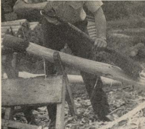
Figure 3.—Round timbers must be peeled before they are treated. Hand tools such as a spade will make this work easier.
