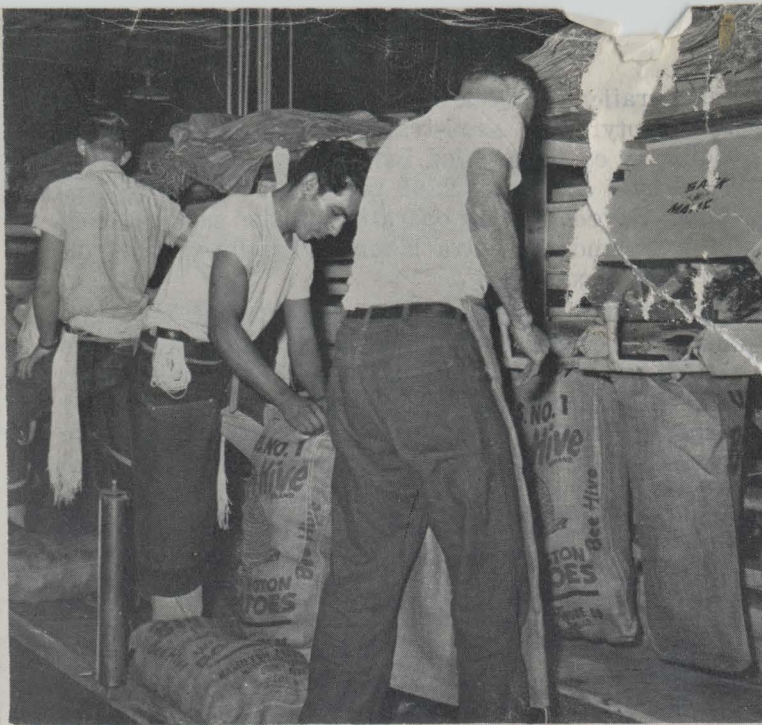
Figure 23—Filling device shuts off when sack reaches 100 pounds. Weighing operation eliminated.
