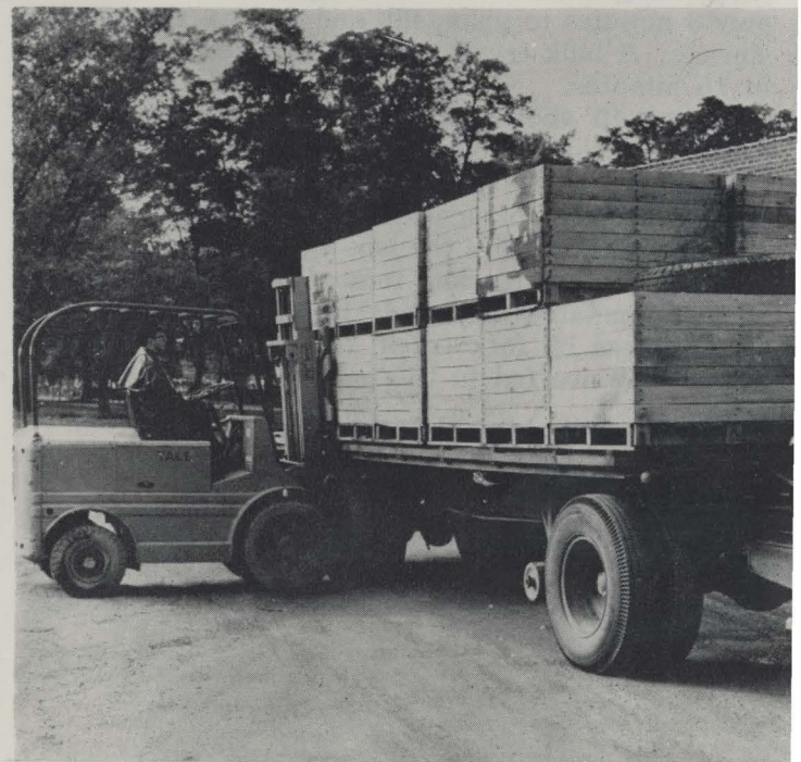
Figure 21—Fork lift unloads bulk boxes at plant. No hand labor necessary.
