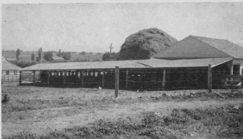
Figure 10.—The shelter provides protection for the manger and a dry feeding floor for the cattle.
