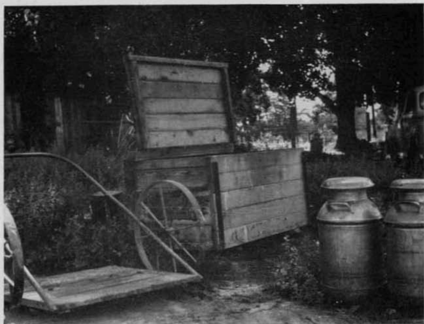
Figure 25.—Plank construction may be used for a 6-can yard or roadside tank. (Plan .845-20)
