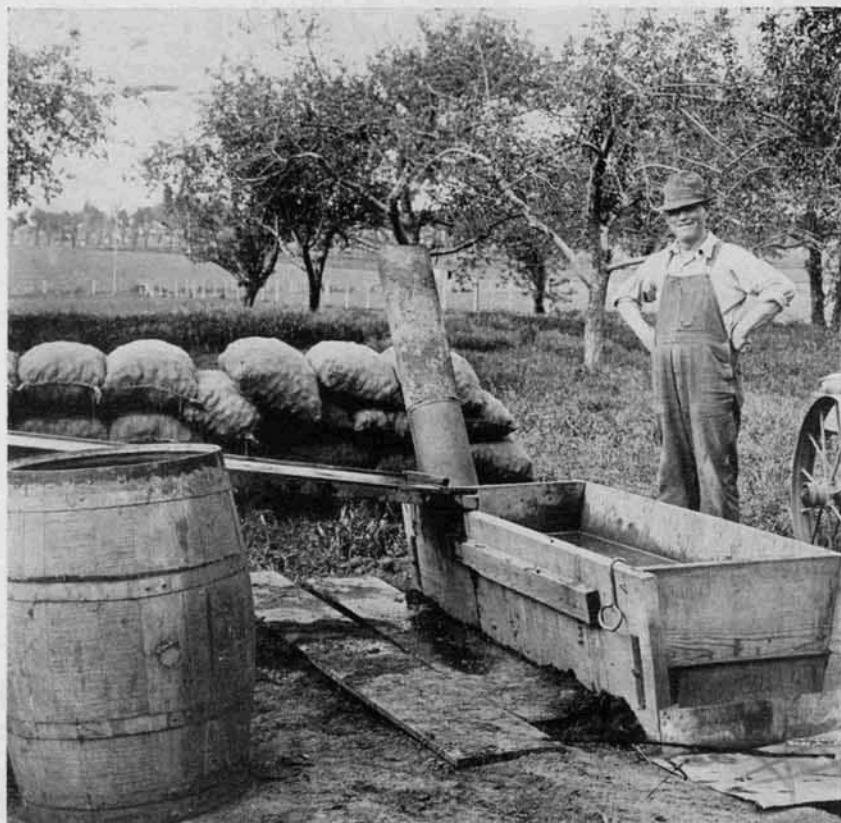
FIGURE 17.—One type of tank used in heating formalin solution. Plank sides, metal bottom, placed over hole in ground.
