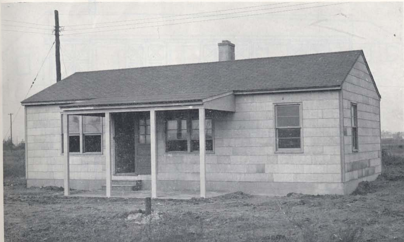
Three-bedroom farm house built from panels and other material taken from a two-story family dwelling unit at Niagara Falls, New York.
