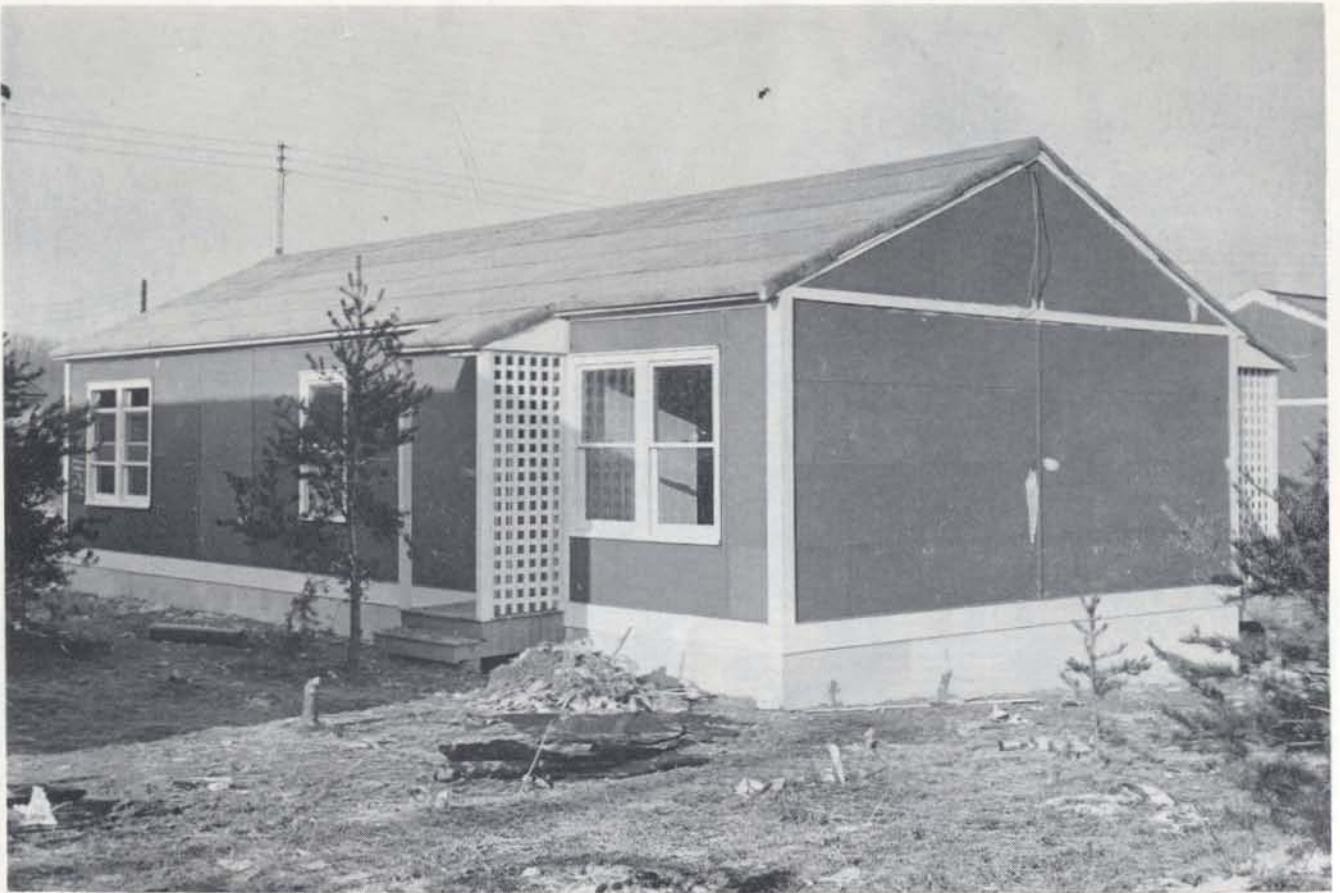
Toilet and shower unit built with panels and other materials from F.P.H.A. war housing units.
