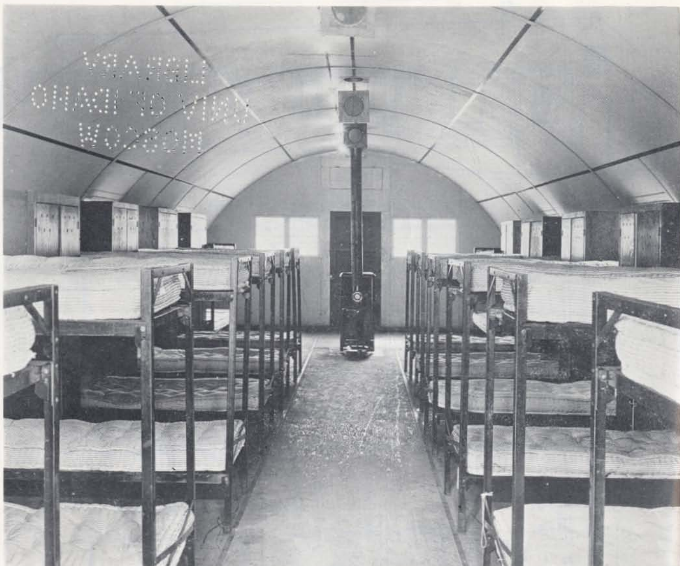
"Quonset 20"—48' long, in use as living quarters. This unit contains 14 double deck bunks and is lined and insulated for maximum comfort and livability.
