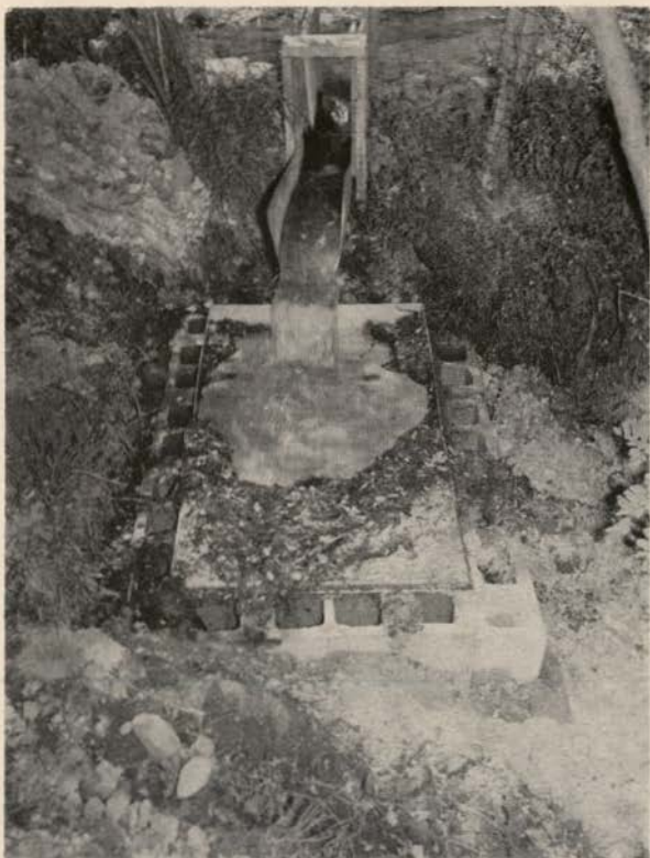
Figure 10. — Screen used in removing trash from irrigation water.
