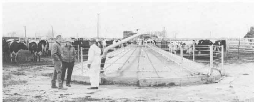
Figure 2. At least one manufacturer distributes glass-lined steel tanks of 20,000 and 34,000 gallons capacity. Cast-in-place reinforced concrete tanks are very satisfactory.
