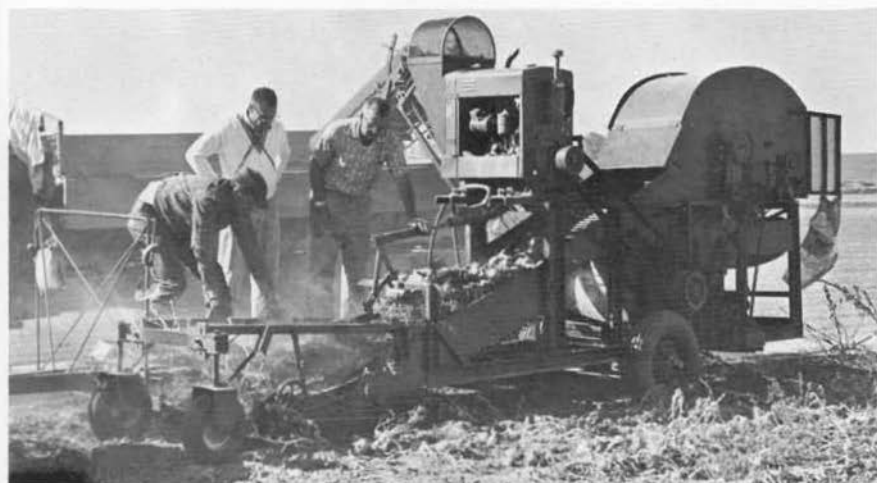
Figure 3. The Air-Flo onion harvesting machine used for machine-topping of the onions.
