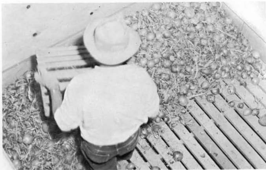
Figure 2. Slatted construction of the bin floors.
