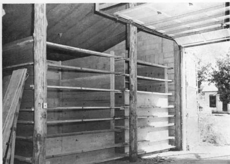
Figure 1. The arrangement and construction of the 8 x 8 x 10 foot bulk bins used for storage during the experiments.
