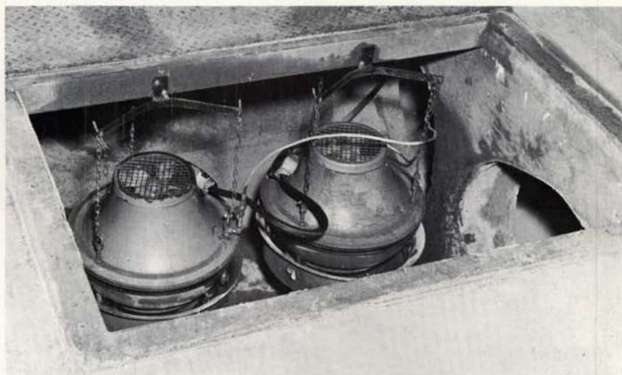
Fig. 4. A centrifugal-type humidifier in an air distribution duct.
