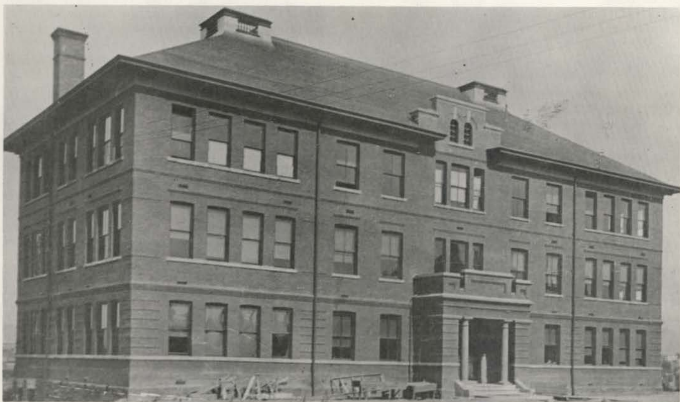
Fig. 7. Morrill Hall was the first Agriculture Building, constructed in about 1907. (#1-66-1, Historical Photograph Collection, University of Idaho Library, Moscow, Idaho.)
