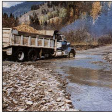
Limited traffic on this improved ford crossing has minimal impact on the stream bed and on sediment production.
