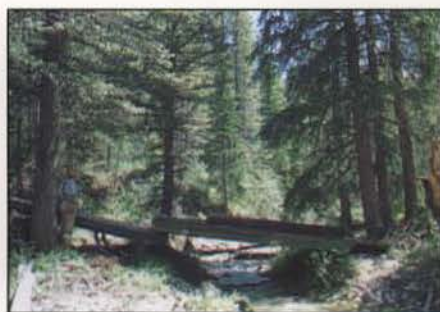
A portable railroad flatcar provides access across streams less than 10 feet wide with minimal disturbance to stream banks or bed. (Stream Channel Alteration Permit may be required.)
