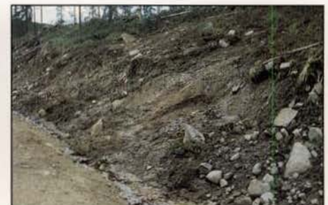
Preventive maintenance can reduce the need for culvert cleaning. In recently logged areas, floatable debris should be cleaned from drainage ditches that direct water to culverts.
