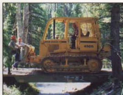
Along with the portability, this temporary bridge is strong enough for all harvesting activities.
