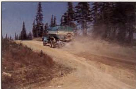
Road surfaces can be protected with the use of water or chemicals. Significant amounts of road surface can be lost as dust, and dust abatement materials serve to decrease rutting. However, they can be pollutants and caution should be used in their application near streams or drainages.
