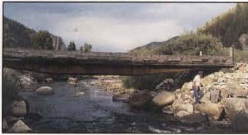
Railroad flatcars can provide a low cost alternative to conventional bridge construction.
