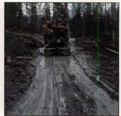
Because roads receive heavy use during logging, be aware of early signs of damage. Serious damage to road surfaces starts with excess water. Standing water is a sure sign of road drainage problems. Ruts indicate that road strength is deteriorating.
