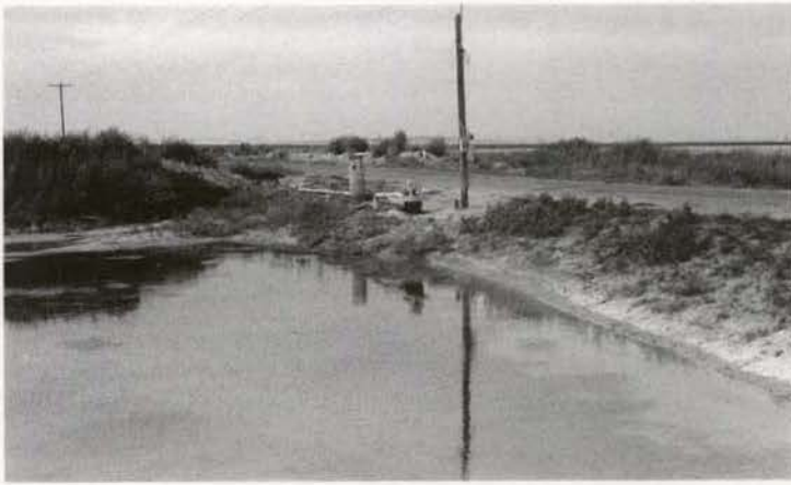
Tailwater Reuse System with storage pond and pump.
