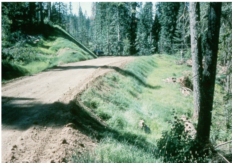
Establishing vegetation on exposed soils stabilizes erodible areas and helps prevent sediment and nutrients from entering water bodies.
