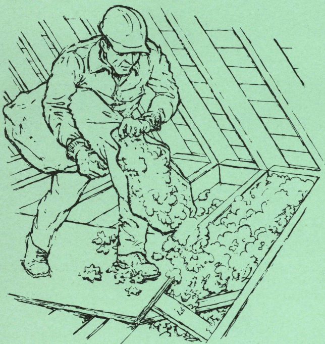
Fig. 2. Loose-fill insulation should be poured into place.
