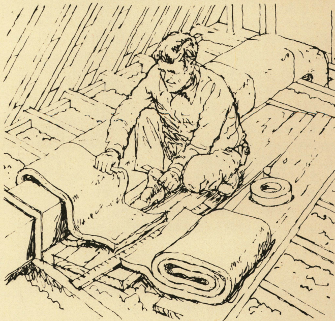
Fig. 4. Insulate heating and cooling ducts which are exposed in attics and crawl spaces.
