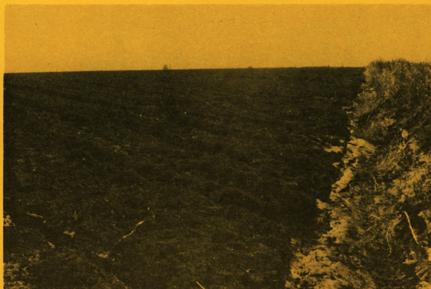
Fig. 1. A rounded or convex field end is a clear sign of soil erosion. This problem needs to be corrected to avoid further damage.
