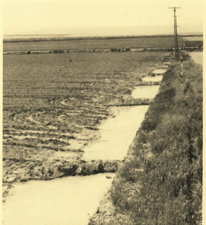
Fig. 1. A buried drain erosion and sediment loss control system operating during the first irrigation after installation.
