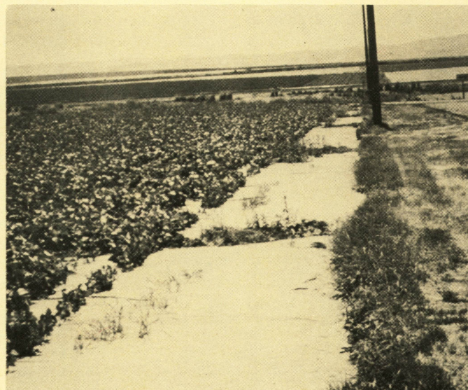
Fig. 4. The same tailwater ditch and sediment basin area shown in Figs. 1 and 3, after four irrigations. The tailwater ditch is filled with sediment, and the convex end problem is corrected.
