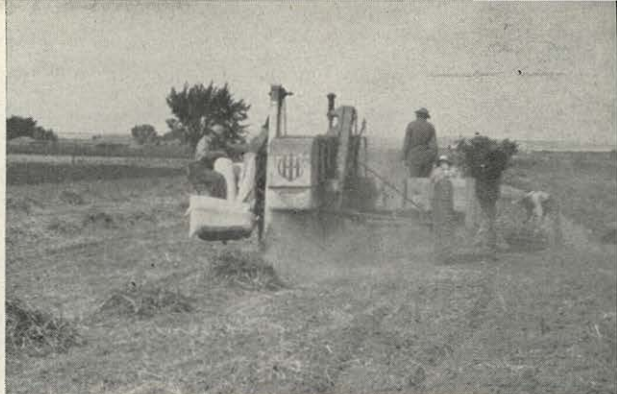
Fig. 10—Threshing carrot seed. Note at right how windrows of roots have been laid out on ground which has been freed of weeds by disking. This not only reduces the amount of weed seeds which find their way into the seed bags, but also reduces loss of carrot seed because the pulled plants lay flat, and hence are not so easily picked up by the wind prior to threshing.
