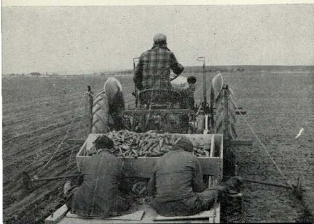
Fig. 8—Showing carrot planting sled and its manner of use.
