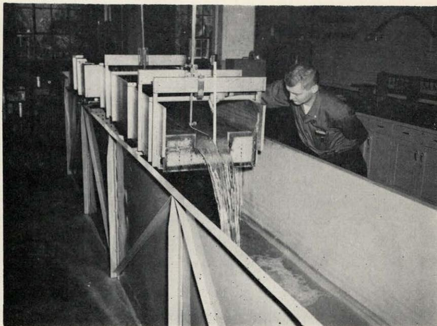
Figure 3.—Gage reading being taken on contracted weir.
