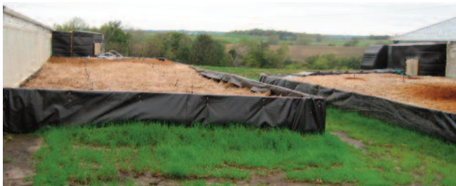
Figure 6. Horizontal biofilter. Photo by Lide Chen.
