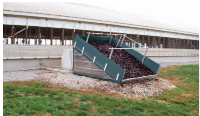
Figure 3. Open-bed, slant-cell biofilter with a sprinkler water supply system. Photo from odorcell.com. Used by permission.
