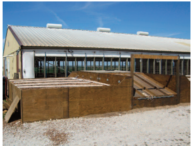
Figure 2. Open-bed biofilter with a PVC pipe water supply system and a bypass louver. Photo courtesy of Dr. Steven Hoff, Iowa State University.
