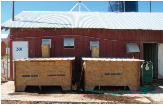
Figure 4. Outside view of a closed-bed biofilter. Photo by Lide Chen.
